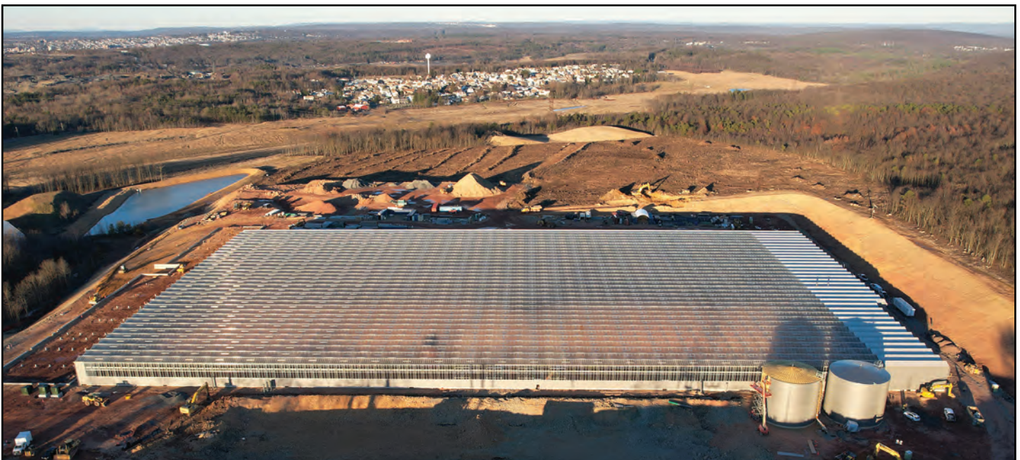
Construction is nearly complete on Little Leaf Farms first of six greenhouses in the McAdoo Industrial Park. It will be the largest greenhouse of its kind in the United States.
