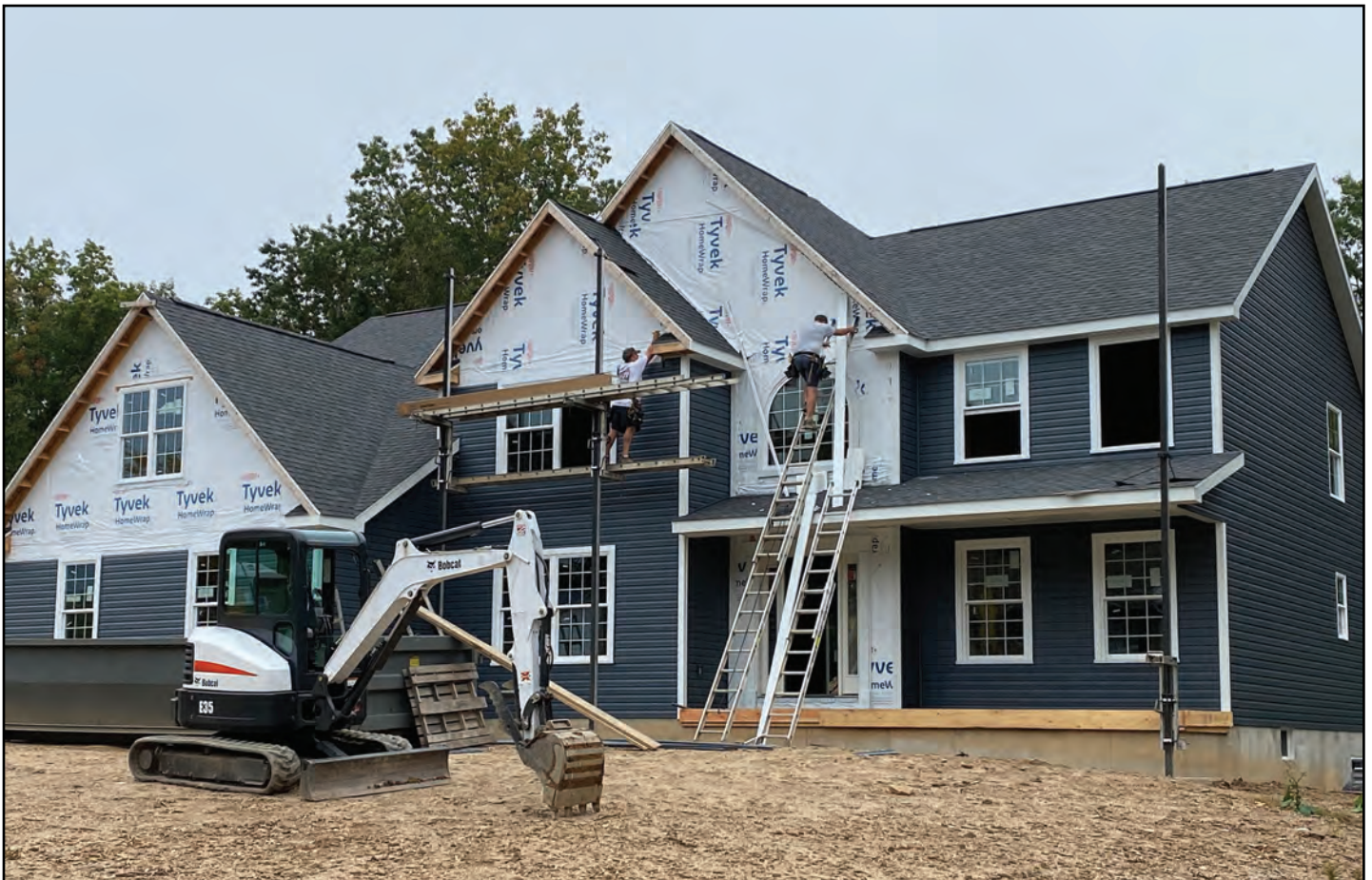
New construction can be seen throughout Greater Hazleton especially in the many housing developments.
