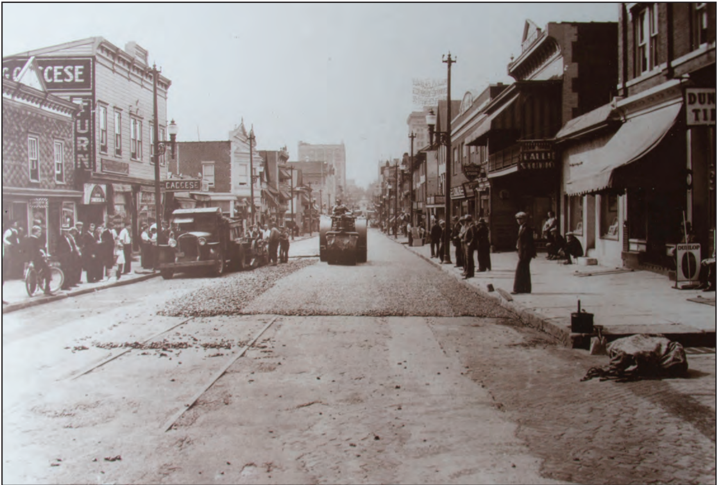
Hazleton residents look on as workers pave Wyoming Street. Today, the street remains one of the main thoroughfares leading to downtown Hazleton.
