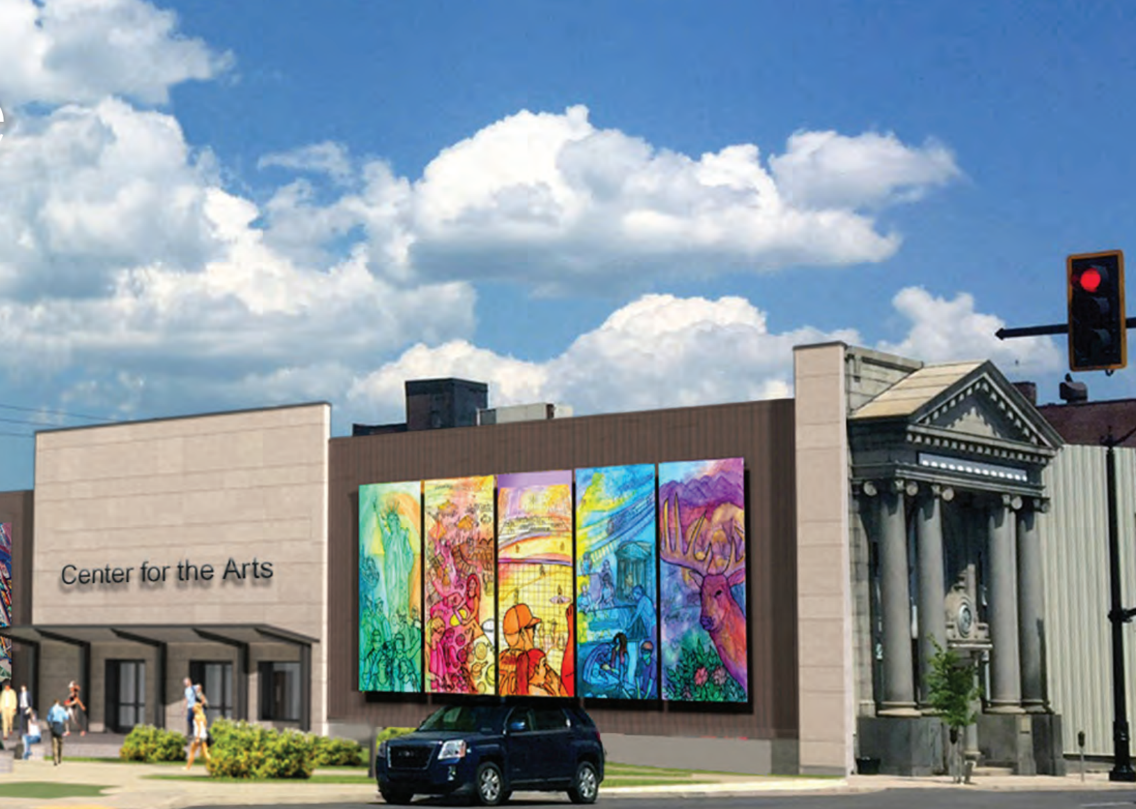
Work is underway to convert the former Security Savings and Loan building on Broad Street into a new Center for the Arts
